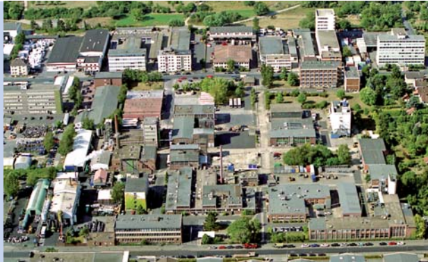
The aerial view shows the impressive extension of the R & D Center
